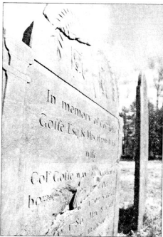
Using an epoxy and specialized tools, a local conservator last week repaired the gravestone of John Goffe, founder of Bedford. Goffe's gravestone broke into pieces 20 years ago. Goffe, buried in the Old Bedford Cemetery, died in 1786.
